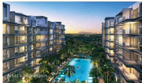
Hedges Park (under construction) • Flora Drive • 501 Units • Expected Date of Vacant Possession: 30 Jun 2015
